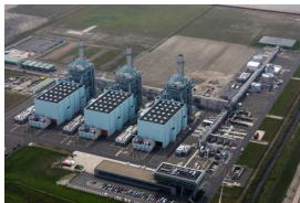
Gas-fired power plants
